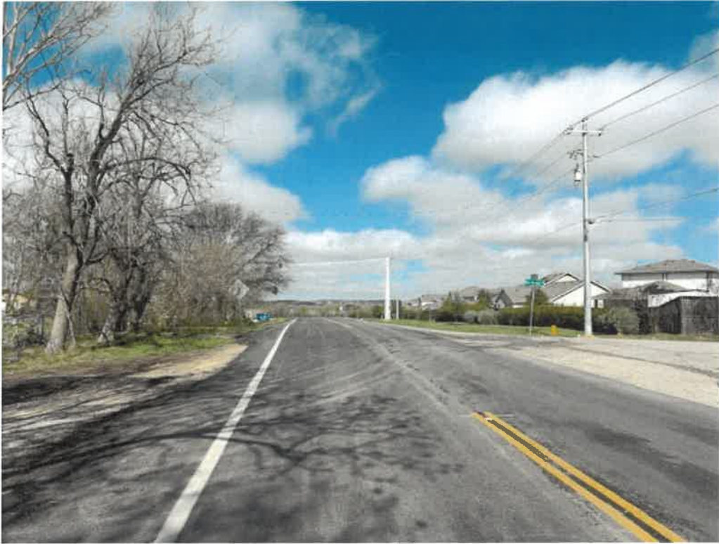
TYPICAL VIEW WEST ALONG FM 812
