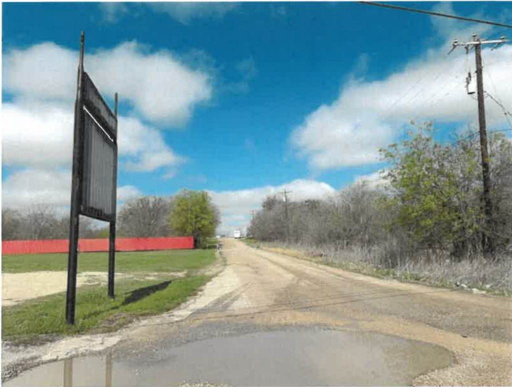
TYPICAL VIEW OF THE SUBJECT PROPERTY FROM US HWY 183
